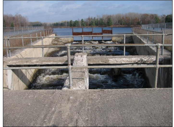
Formation of sinkholes along the dam spillway and deteriorating concrete shows sign of excessive damage and failure potential (2018)
