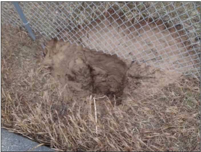
Formation of sinkholes along the dam spillway and deteriorating concrete shows sign of excessive damage and failure potential (2018)
