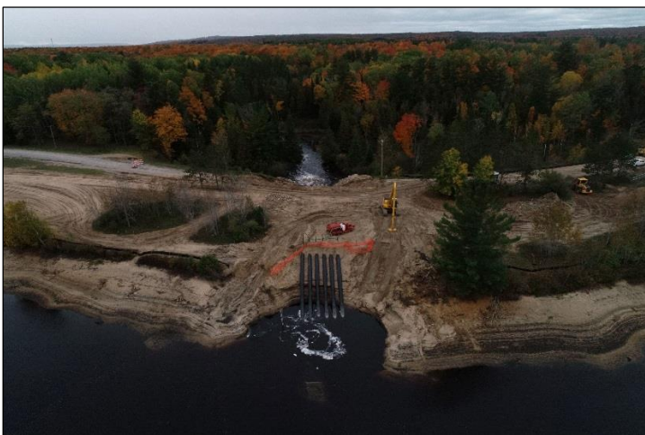
Drone photos of Lake Kathleen Impoundment, Dam, and Dewatering System (Sept 2018)
