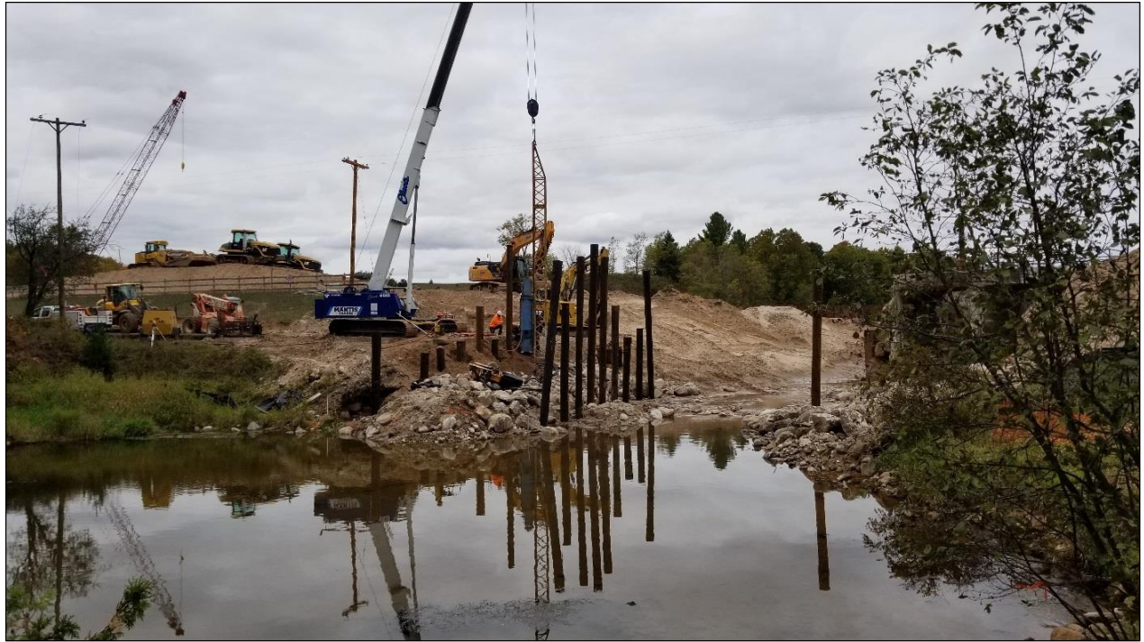
Woodland Rd. Project During Construction – pile driving, deck placement, and paving 2018 (above and below)
